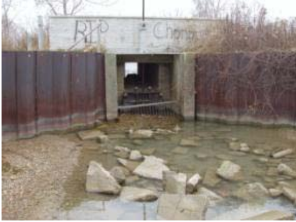
View of the Structural Barrier to the Detroit River
