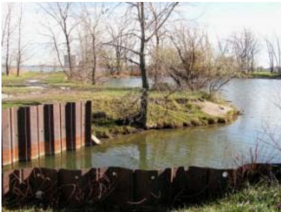
View of the Connection with Detroit River
