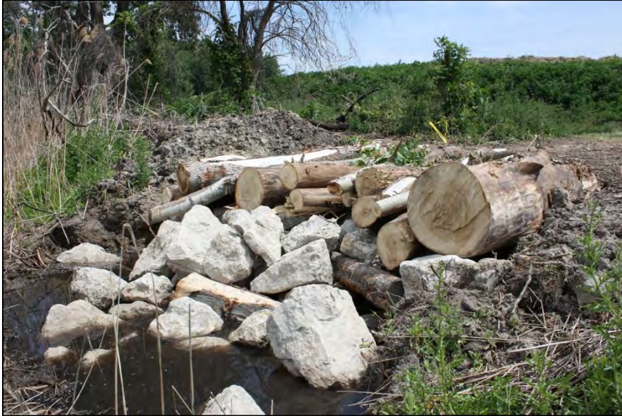
Photo 22. Hibernacula such as this one that is under construction can be created using simple materials such as logs and riprap.
