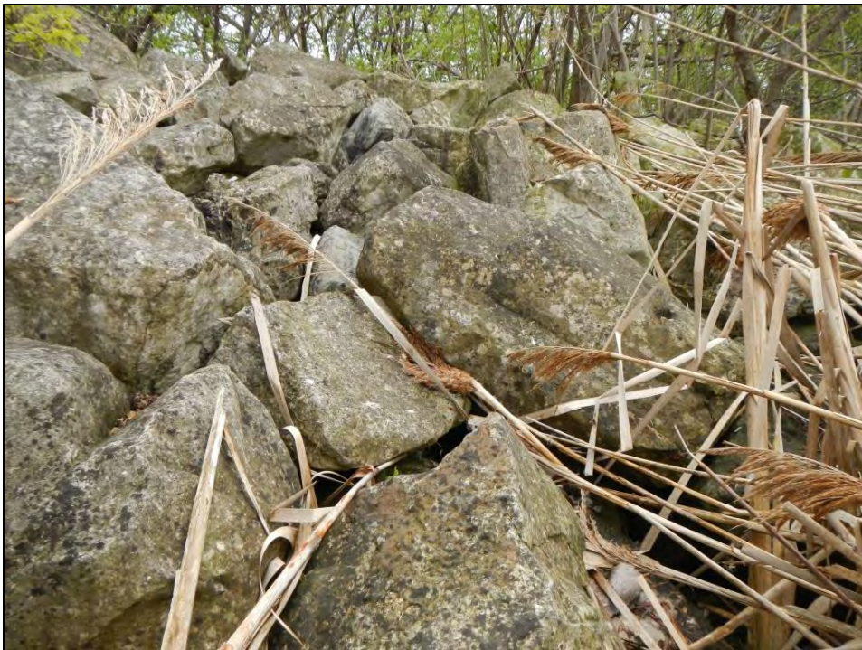
Photo 12. Large rocks along riprap dikes on Stony Island. Filling in portions of these dikes with smaller gravel and cobble will facilitate easier movement of herpetofauna including turtles.
