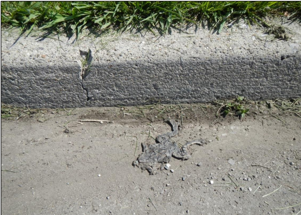
Photo 32. Curbs can act as barriers to herpetofauna. Installing rolled curbs or eliminating them all together can help prevent roadside mortalities.
