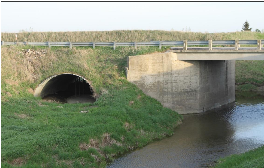
Photo 30. Creating crossing structures such as this one can provide passage for both aquatic and terrestrial species while minimizing risk of road mortality.
