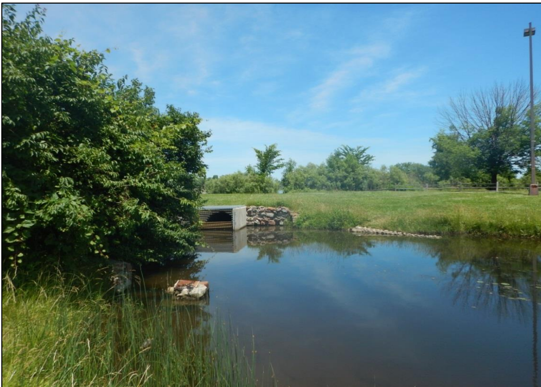
Photo 6. Current hydraulic connection between LO and the Blue Heron Lagoon.
