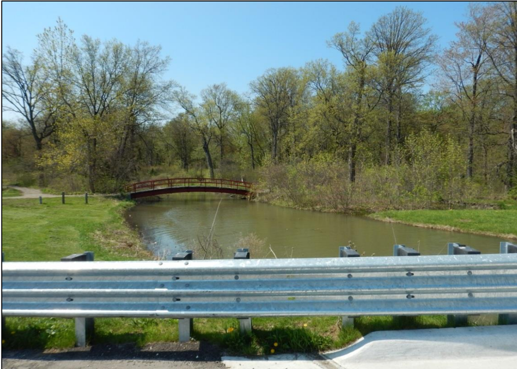
Photo 5. View north from the Woodside Drive bridge over Nashua Canal.
