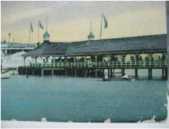
PHOTO 6. SUGAR ISLAND NORTH DOCK
