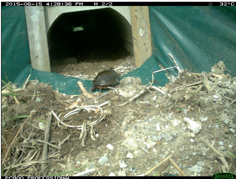
Photo 28. An example of a culvert in use: a Painted Turtle using a under-road culvert. Photo credit: “More aquatic wildlife culverts for Long Point Causeway” by LPCIP News, 2015.
