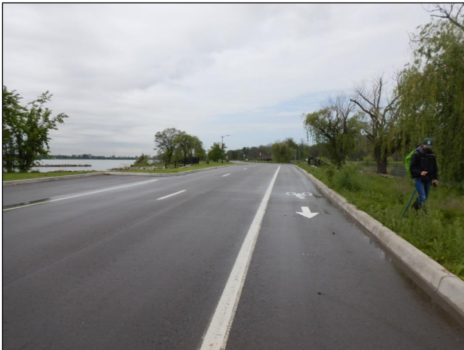
Photo 26. High curb observed along The Strand Road creating a barrier to herpetofauna movement.
