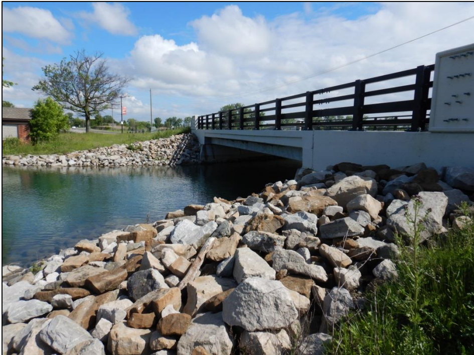
Photo 8. Riprap made up of large rocks on the sides of a culvert connecting Lake Okonoka to Blue Heron Lagoon. This area supported several Northern Water Snakes.
