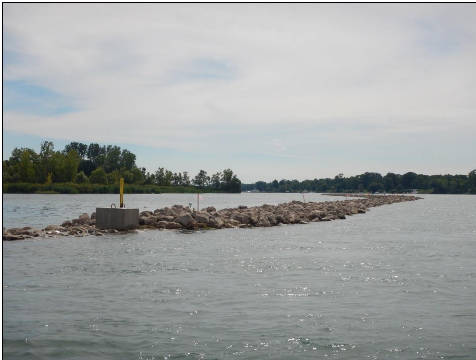
Photo 22. Newly constructed replacement shoal on northern portion of Stony Island.
