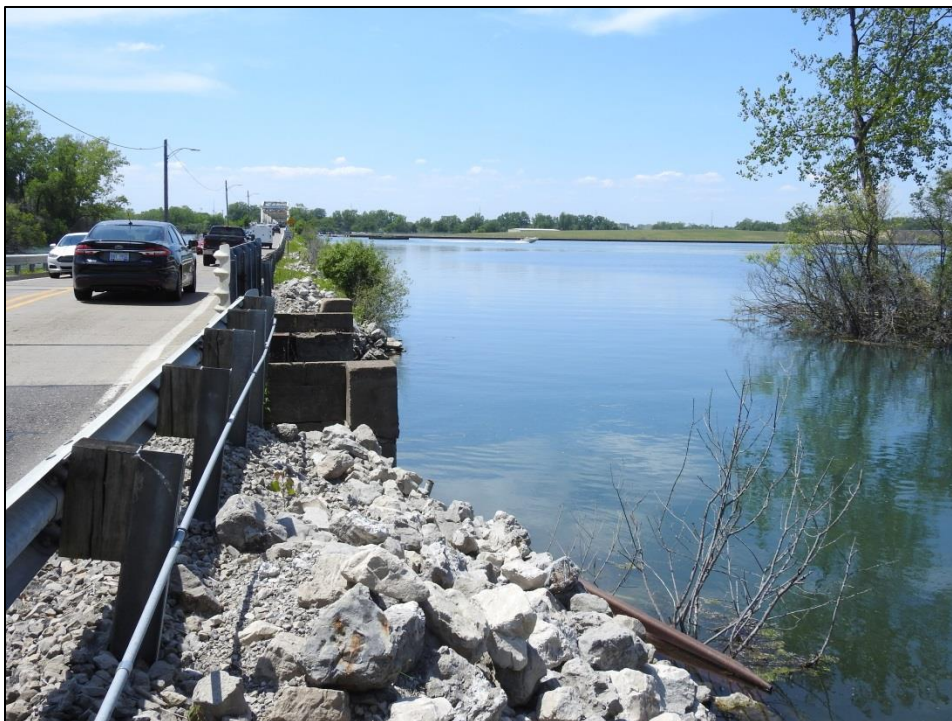
Photo 9. Small interstitial rocks should be incorporated between larger rocks to prevent turtles from getting stuck in gaps.
