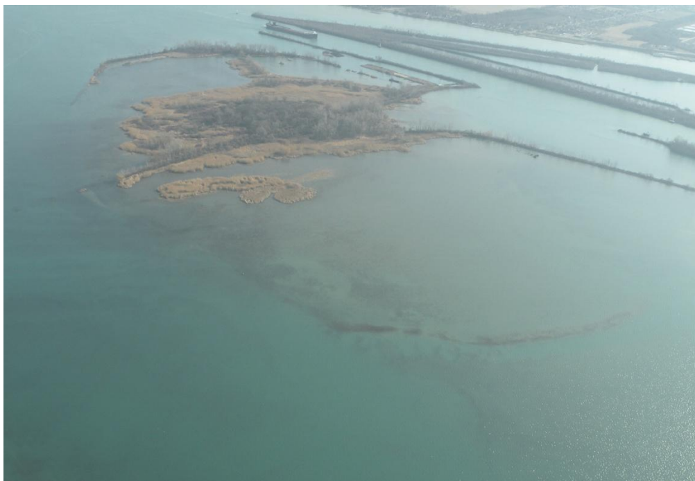
Figure 15 – Aerial Photograph of Stony Island Showing Shoal Reconstruction Areas
